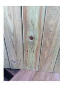
SECURE WITH 9 SUPPLIED SCREWS (3 INTO EACH) FROM INSIDE THROUGH PRE DRILLED AND MARKED HOLES.
